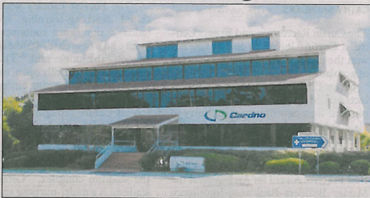
Tenant: Infrastructure consultancy Cardno leases the Bagot Road property.
